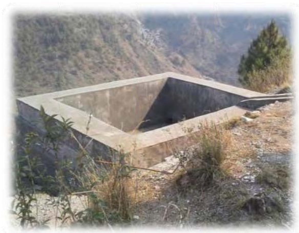
Irrigation Tank, Badeth village (Revati Valley)
