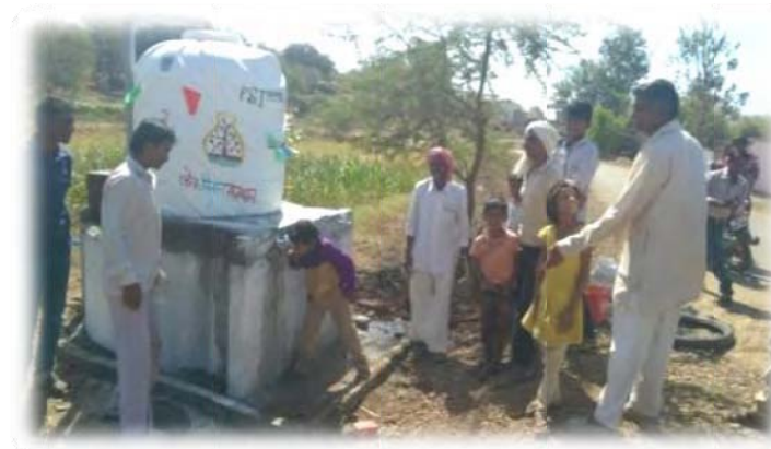
Drinking water supply tank in Bankpura village
